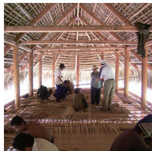
Reconstruction management of vernacular architecture and indigenous technology
