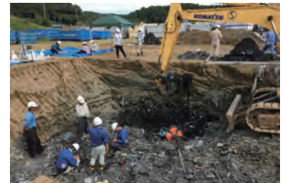
Site investigation at a waste landfill site
